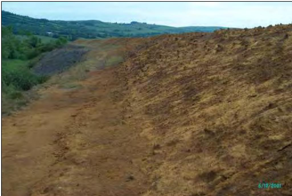
Partially Vegetated Outer Slope on South Side, with Indications of Wind Erosion
