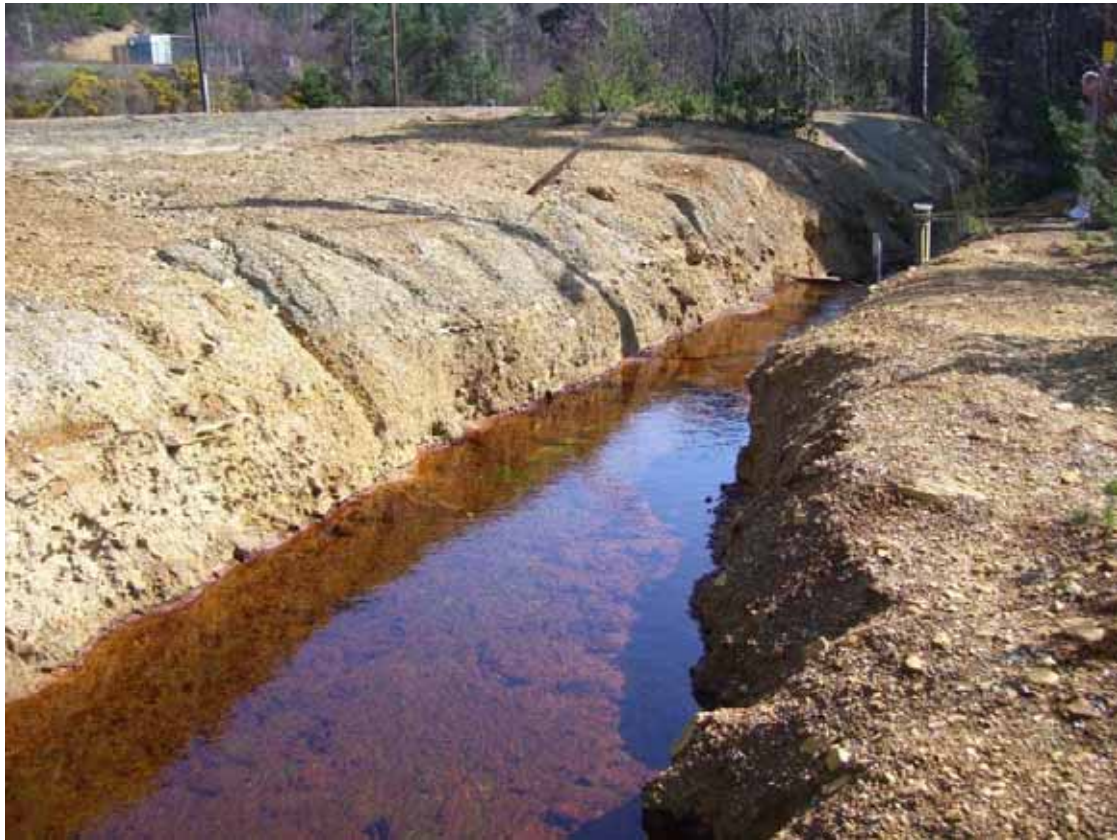
Figure 5-5 Red-brown precipitate in the channel which conveys the Deep Adit discharge from the portal to the Avoca River (April 2007).
