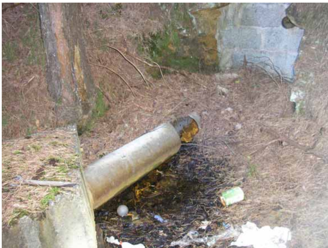
Figure 3-7 Spa Adit showing bulkhead and discharge exiting the break in the pipe (August, 2007).
