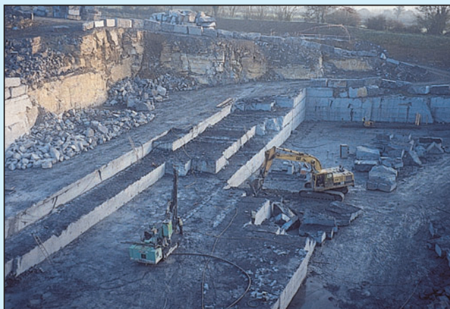
Dimension stone quarry, Co. Roscommon. (Courtesy Feely and Sons Ltd.)
