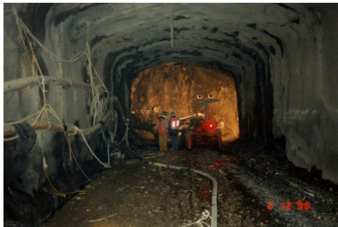
Underground operations at Galmoy
