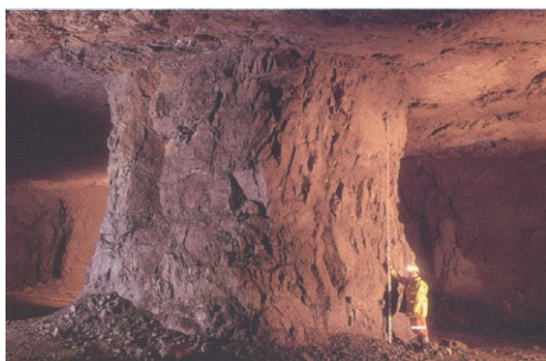
Safety pillar underground
